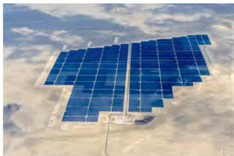
Figure 6. Aerial photo of First Solar's 300-MW PV power plant. Photo from First Solar
